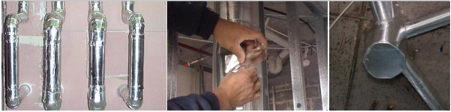
Simply use AGC tape to affix and join Soundlag even around complex bends in pipework.
